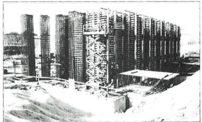
NIF Target Area retaining wall forms and rebar.
